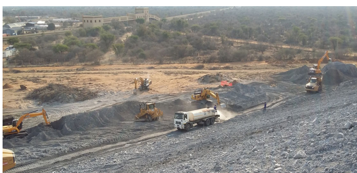
CONSTRUCTION OF THE SLIMES DAM 7 RETURN WATERLINE AND SILT TRAP
