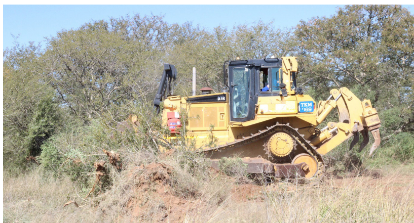
TKM Engineering dozer debushing the Sebele Horse Race Track
