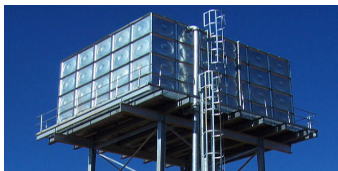
DESIGN, SUPPLY, INSTALLATION AND COMMISSIONING OF 200M3 GALVANISED STEEL (GS) TANK ON 15M STAND IN GOODHOPE VILLAGE INCLUDING A 10KM UPVC PIPELINE IN GOODHOPE & PITSA NE VILLAGES
